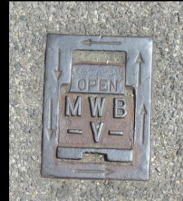
METROPOLITAN WATER BOARD STOPCOCK ACCESS COVER, PORTSMOUTH ROAD, LONG DITTON, 25 JULY 2026
