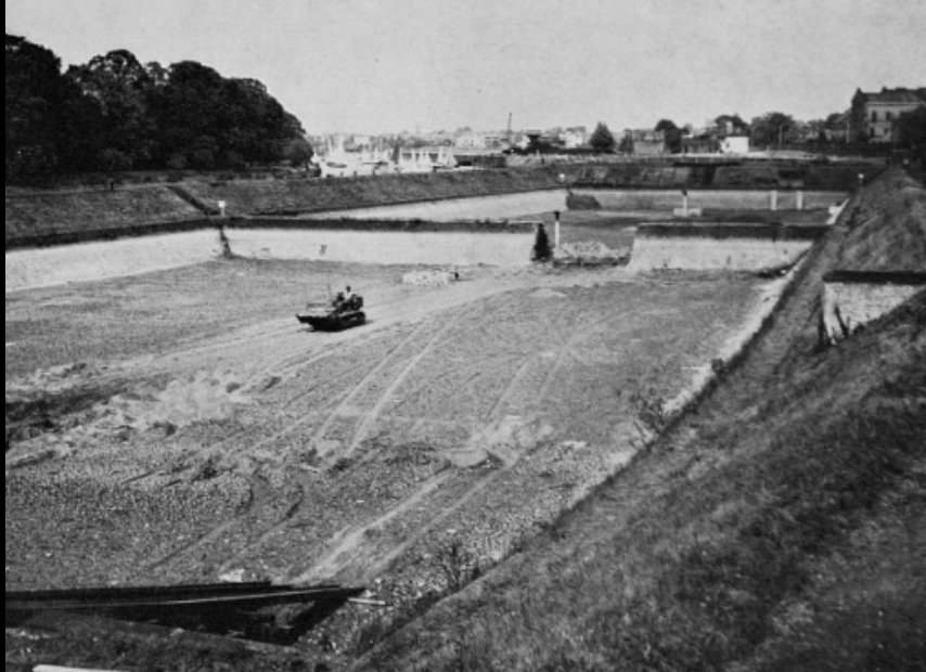
THAMES DITTON MARINA CONSTRUCTION, 1957
