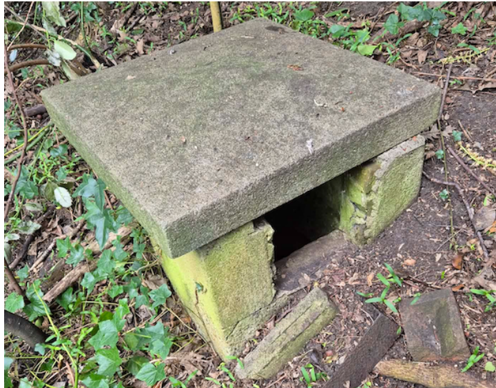
Figure 5. A ventilation shaft for the tunnel? Photograph by Jon Pitman, June 2026
